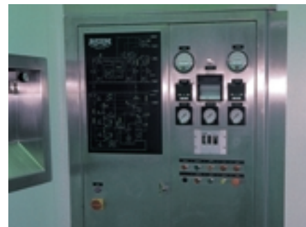
DETAIL OF CONTROL PANEL
